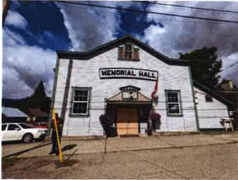
Hall from east
